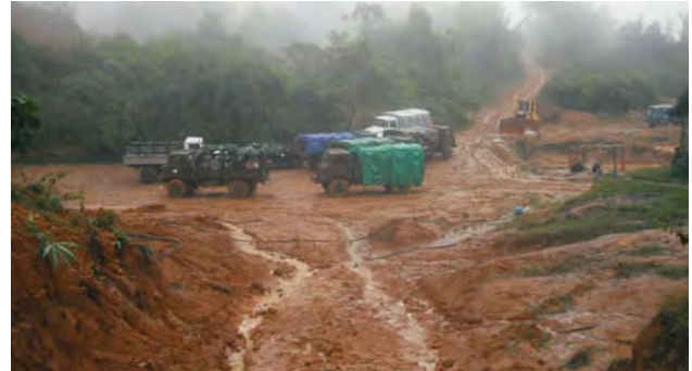
Ban Houay Xai Site conditions
